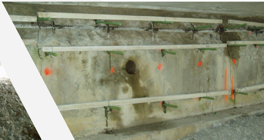
Figure 5 – Dowels and anodes installed
