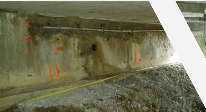
Figure 4 – Spall removal
