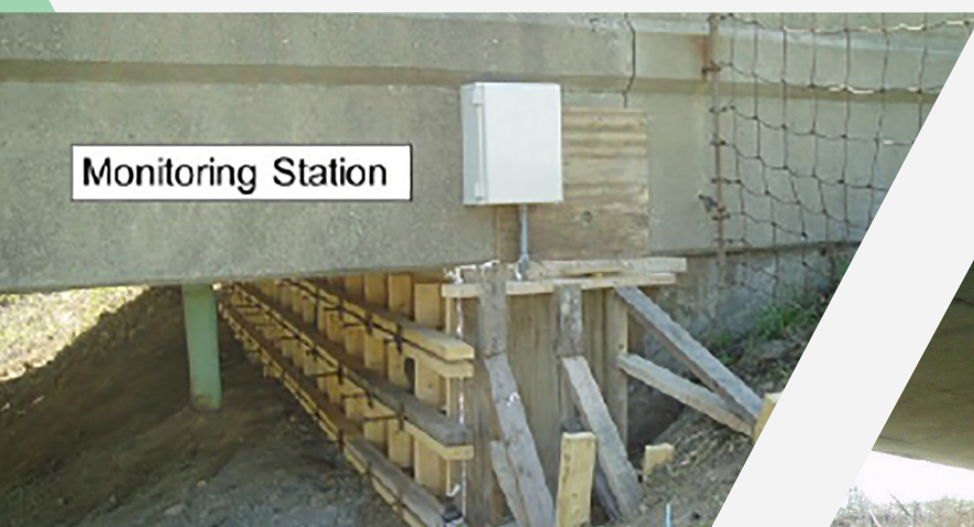
Figure 6 – Formwork and monitoring station prior to pumping SCC
