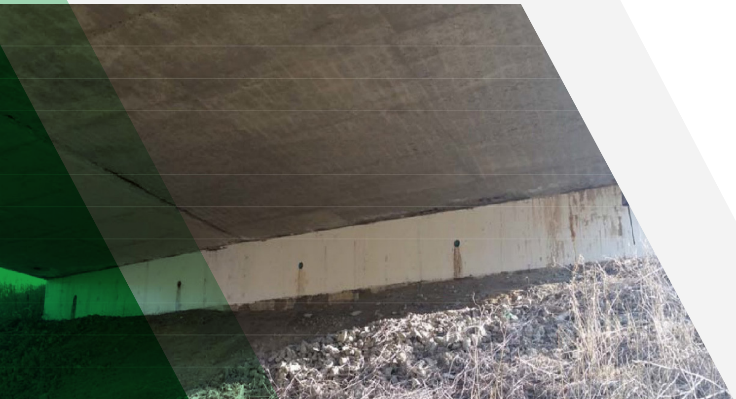
Figure 8 – Abutment of I-75 Bridge over Kirkwood Road (mm 87) in 2022 (Note efflorescence from leaking joint and weep holes)
