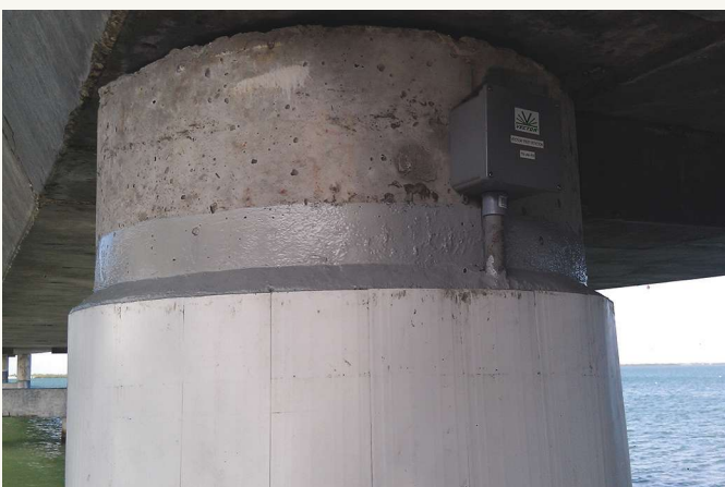
Figure 7. Self-activated anodes inside modular PVC formwork.
