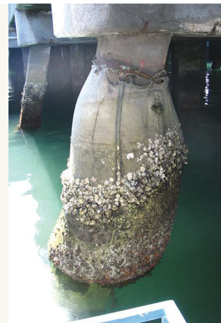
Figure 2. Fabric form jacket with concrete fill.
